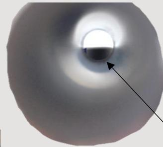
Edge of white cap should be in the center of the t-riser
